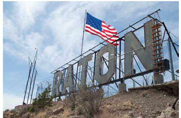
The RATON sign is one of 12 contributing structures in the district. At left is the "Star of Bethlehem" first displayed as a Christmas decoration. Both structures were built in the 1930s. photo: John Murphey, who wrote the National Register nomination.
